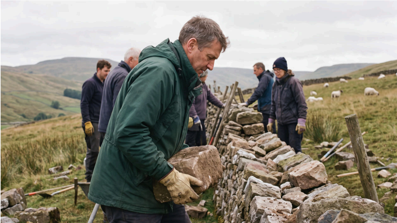
Colleagues rebuilding a dry stone wall in the Yorkshire Dales on a volunteer day.
